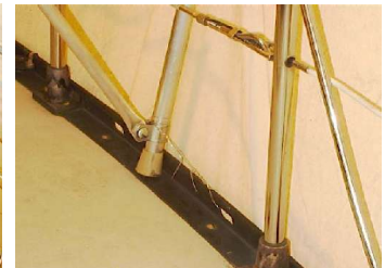
Bracing / Pipe strap tied to toe rail
